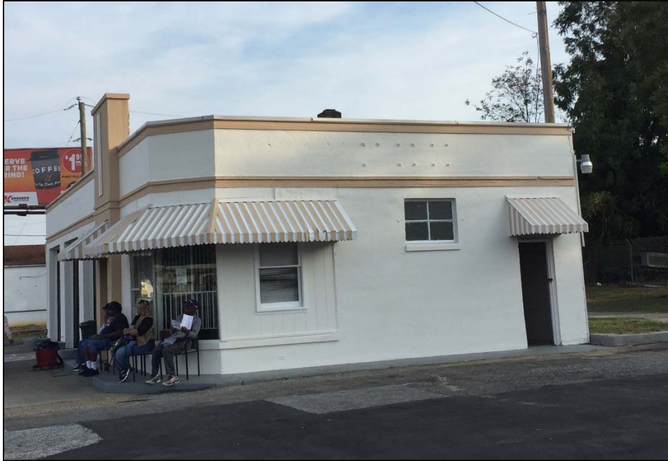
Figure 52. Crossover Service Station.
