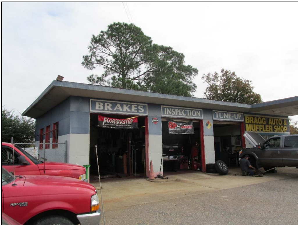
Figure 45. North elevation and service bays.
