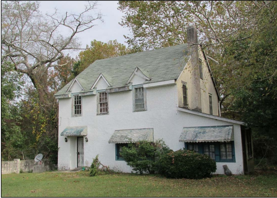
Figure 20. Jesse Williams House, front and south elevations.
