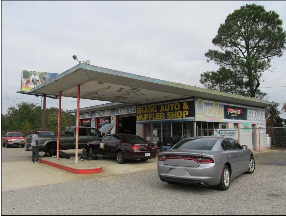
Figure 41. Bragg Auto & Muffler Shop, west and south elevations.
