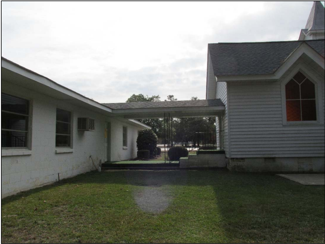
Figure 10. Walkway between Sunday school building and sanctuary.
