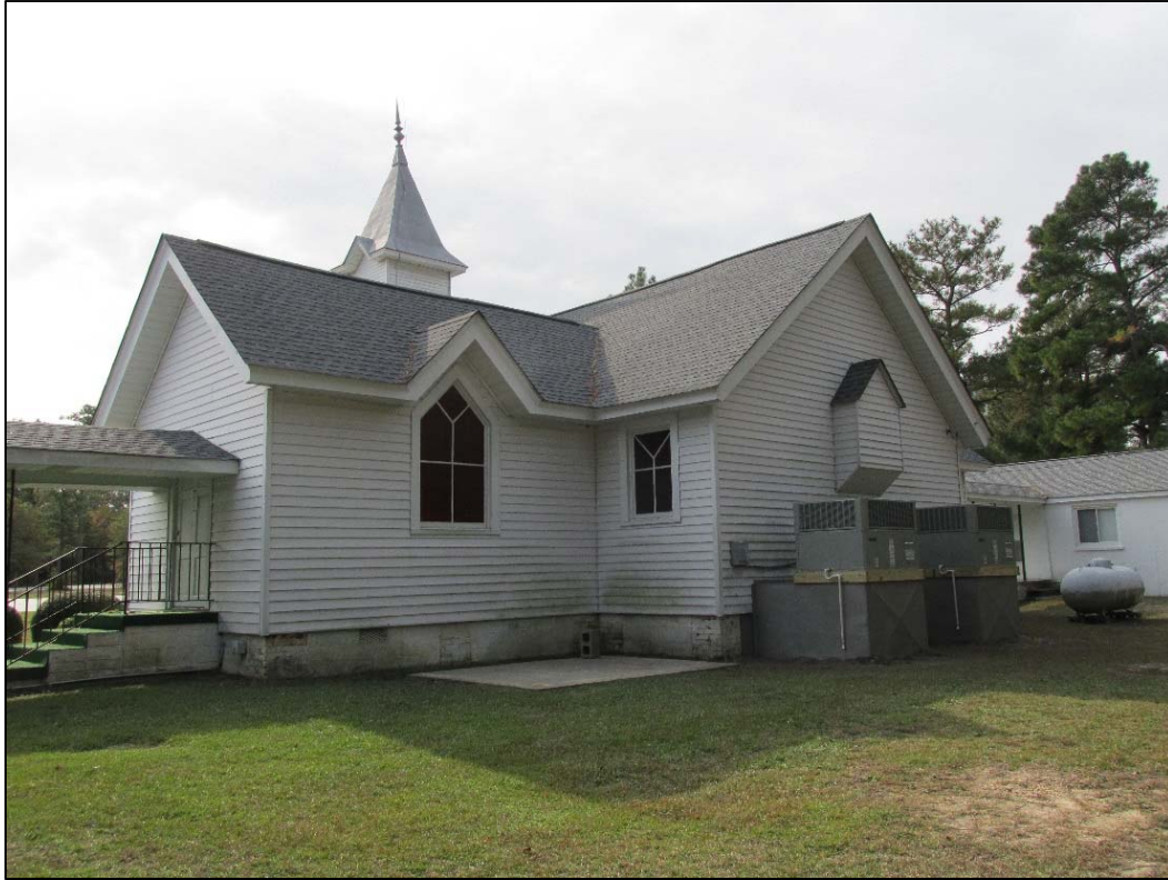
Figure 6. Sanctuary, rear and east elevations.
