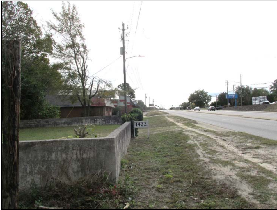
Figure 23. Wall around front yard.
