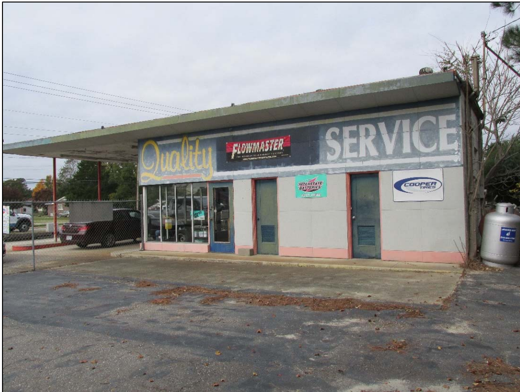
Figure 43. Bragg Auto and Muffler Shop, south elevation.
