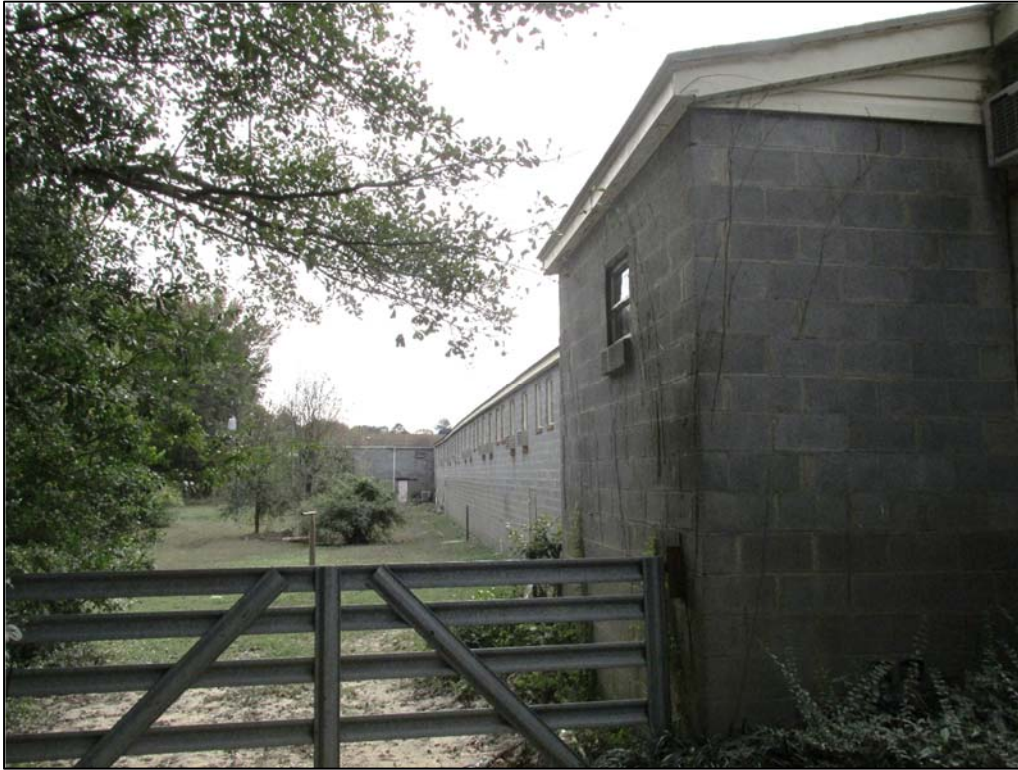
Figure 31. Starlite Motel, rear elevation.
