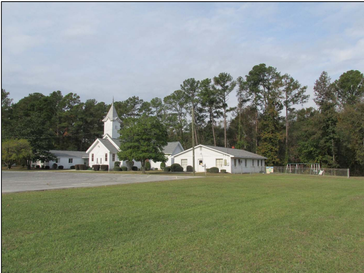
Figure 3. Church of the Covenant, south and east elevations.
