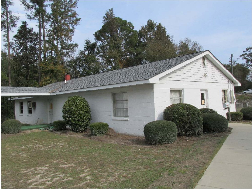
Figure 9. Sunday school building, south and west elevations.
