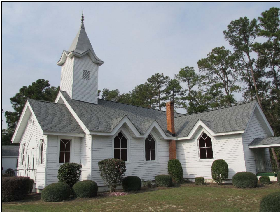
Figure 5. Church of the Covenant Sanctuary, south and east elevations.
